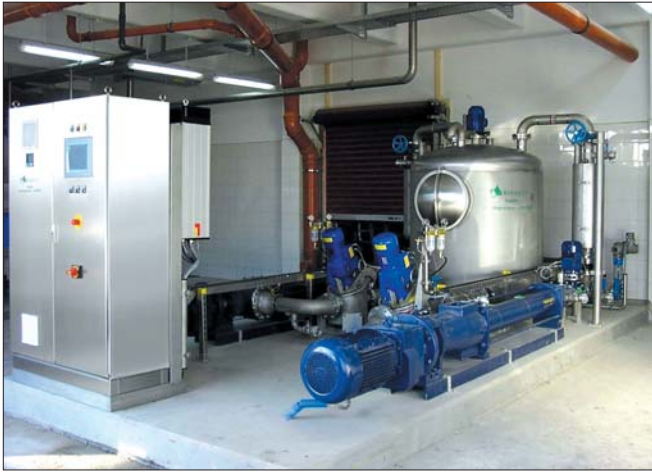
The Crown® solids disintegration system is a U.S. patented cell lysing process that eliminates digester foaming, increases gas production by up to 30 percent, and reduces solids for disposal by 20 percent.
