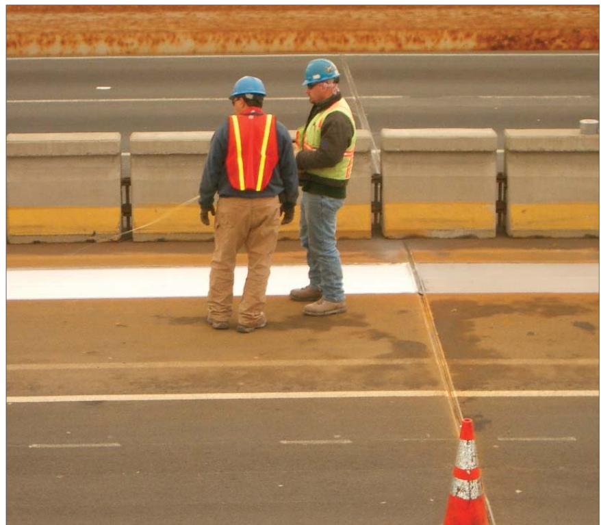
Median barrier weld surfaces are protected by a proprietary primer that protects the weld areas, improves weld quality, and continues to ward off corrosion throughout the years.
