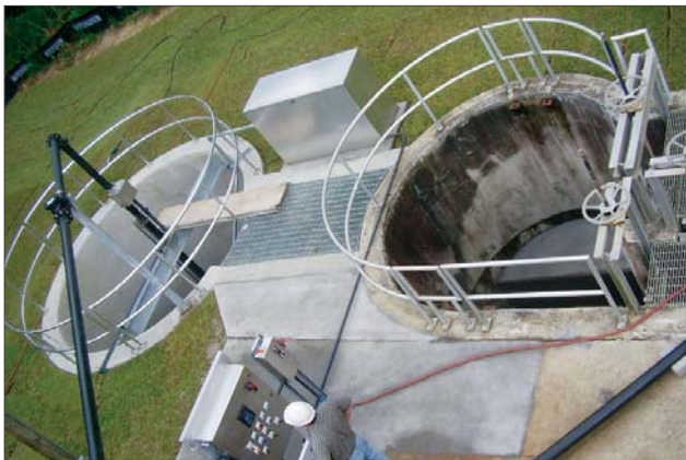
The grit removal system is comprised of the Grit King unit and a grit washer/classification unit. Valving, grit classifiers, grit pumps, dewatering decanters, and control systems are available to provide a comprehensive grit removal package.
