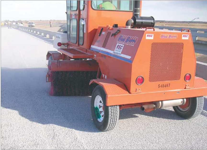
...after which excess aggregate was removed by sweeping.
