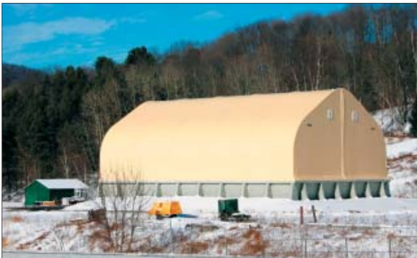
TITAN buildings used for salt storage range in size from 50 ft to 60 ft wide and about 90 ft long.
