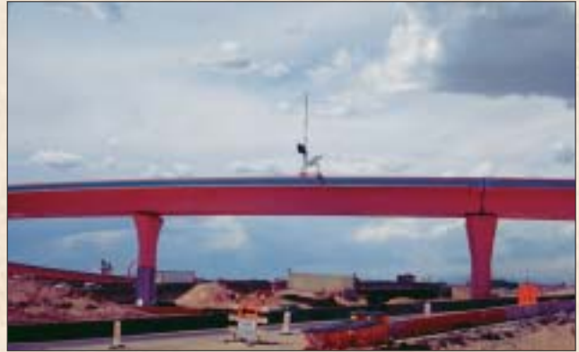
Example of ITS equipment deployed at the Big I.
