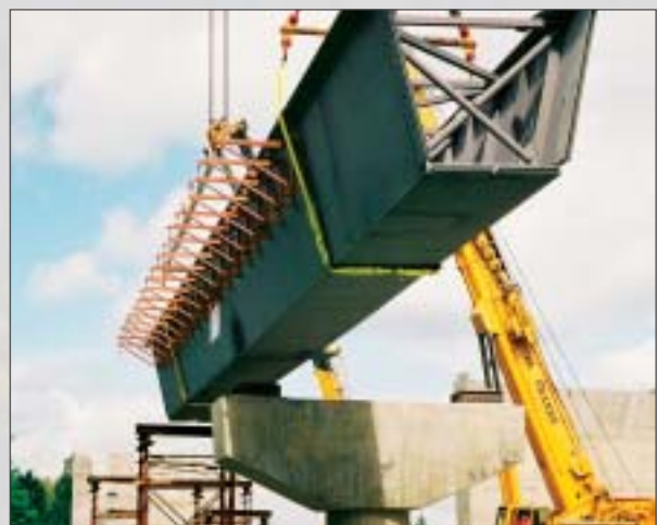
The Crossing Bridge was built using 45 precast concrete U-shaped girder segments that were dropped into place and post-tensioned together.
