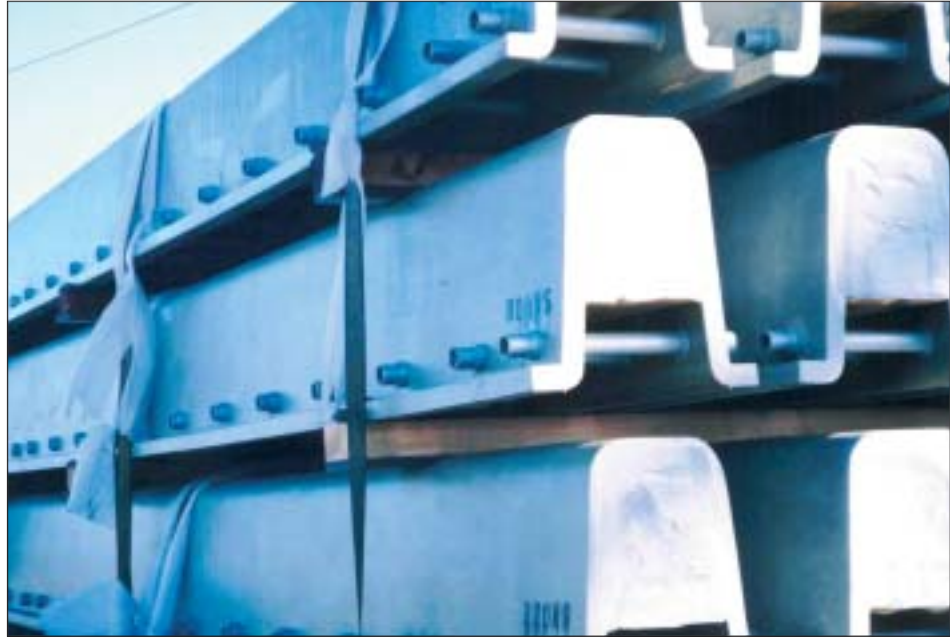
Twelve of the 30-ft beams could be transported on a single trailer. Lightweight foam fills the bottom of the beam's included volume to conserve concrete.
