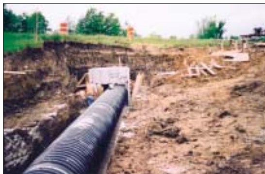
The combination of a corrugated exterior and a smooth interior enable the pipe to provide both strength and optimum hydraulic capacity.
