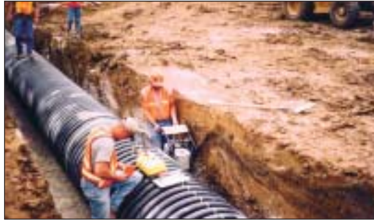
Specially engineered polymers enable the HDPE pipe to meet standards issued by the American Association of State Highway and Transportation Officials.
