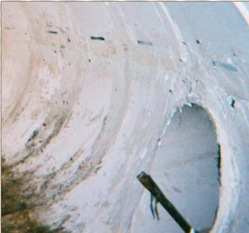
The 90-degree bend with a 30-in. side connection after repair.
