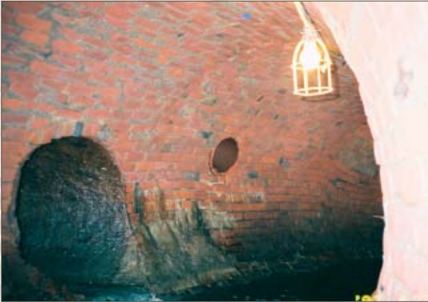
The 90-degree bend with a 30-in. side connection before repair.
