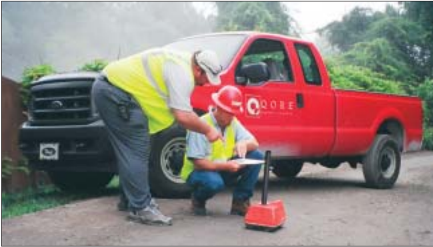
Quality control consists of nuclear density readings as well as before and after sampling involving gradation and AC-extractions back at the laboratory.
