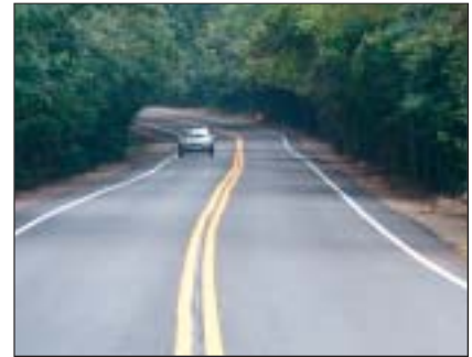
The newly rebuilt Riverside Road has an added shoulder made from reclaimed asphalt pavement that was taken from another phase of the project. The additional platform width provides bikers and bicyclists a smooth path to share with cars.
