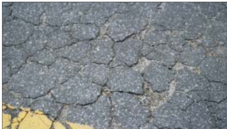
Once an aged asphalt pavement is alligatorized to this extent the reclamation process provides a new 20-year life cycle at a fraction of the cost of conventional reconstruction techniques.
