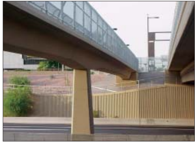
The pedestrian bridges present a slender and elegant appearance, enhanced by sloped abutment faces and tapered pier columns.
