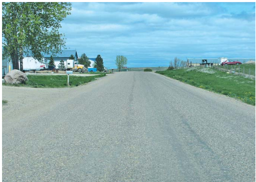
Otta Seal surface near a business that generates heavy truck traffic.
