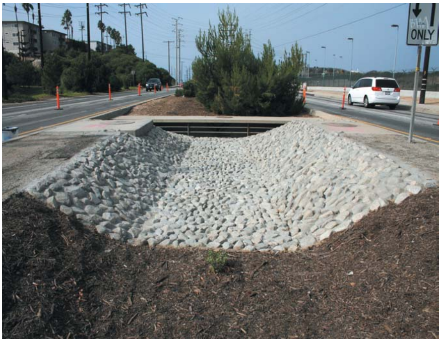
Riprap protects the soil from erosion in front of the storm drain on a median along Imperial Highway in Los Angeles.
