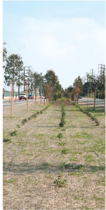
The Imperial Highway Median Stormwater best management practices project treats urban runoff through infiltration trenches and vegetation.
