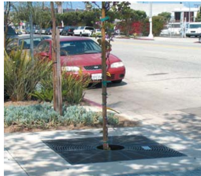
One of seven bioretention filters installed in Venice as part of the grand Boulevard Tree Wells project.
