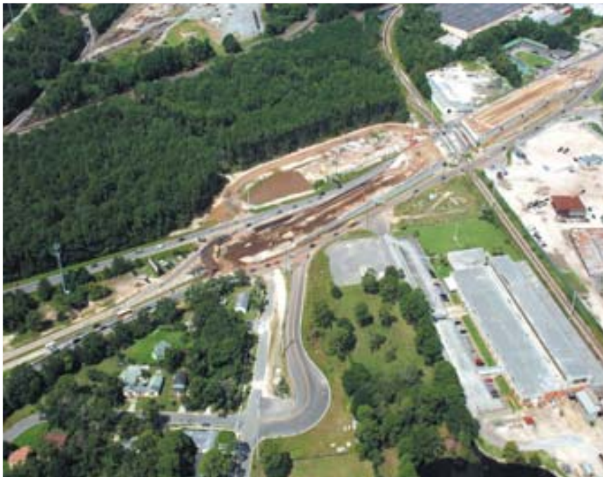
Over a 100 lane-miles of roadway improvements are by far the largest portion of the Better Jacksonville plan, totaling over $1.5 billion of the available $2.25-billion comprehensive growth management program. Photo courtesy of www.aerophoto.com.
