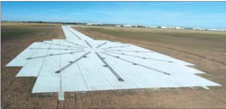
Aerial view of the Compass Calibration Pad, which sits in a magnetically quiet zone where an aircraft’s compass can be calibrated at the Newton City/County Airport, just north of Wichita, KS.
