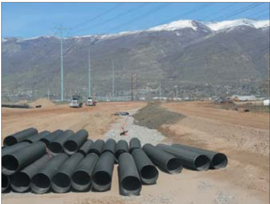
Here, the HDPE drainage pipe awaits installation, a process that is facilitated by its light weight requiring only one- or two-person crews.
