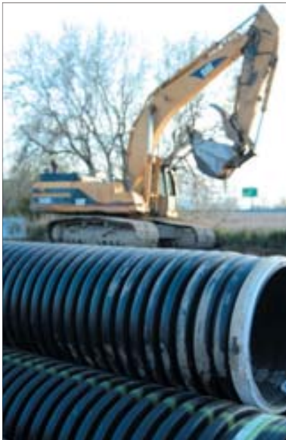
The HDPE pipe features a corrugated exterior and smooth interior for both strength and maximum hydraulic capacity.
