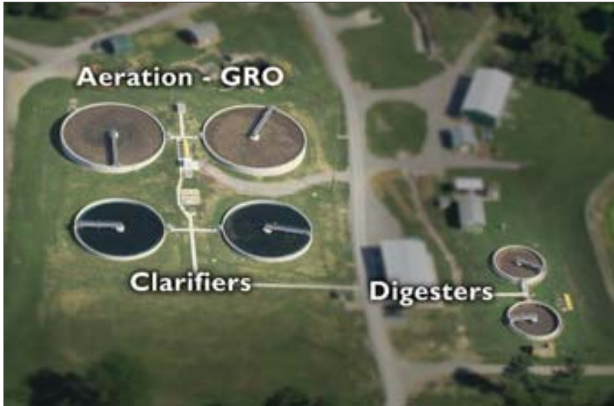
Aerial photograph of DuQuoin's wastewater treatment plant shows the relationship of the aeration tanks, clarifiers, and digesters.
