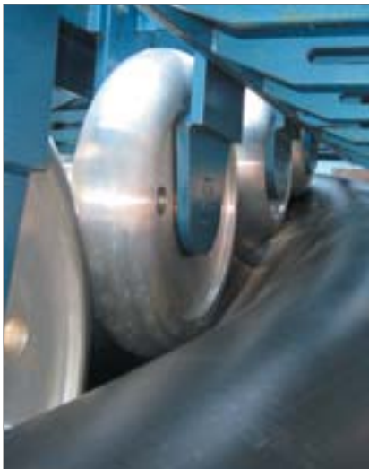
The HDPE pipe is first folded before being banded.
