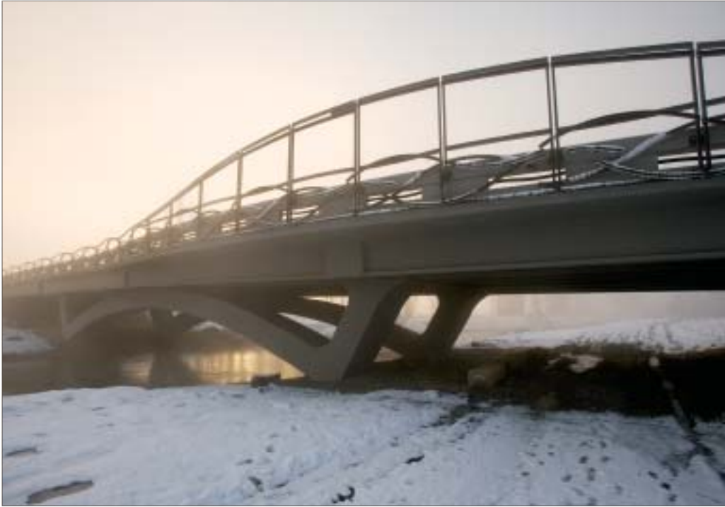
Clear separation of the trail running below from the bridge itself makes recreational activities safer for pedestrians, skaters, and bicyclists. Photo by John Livzey.
