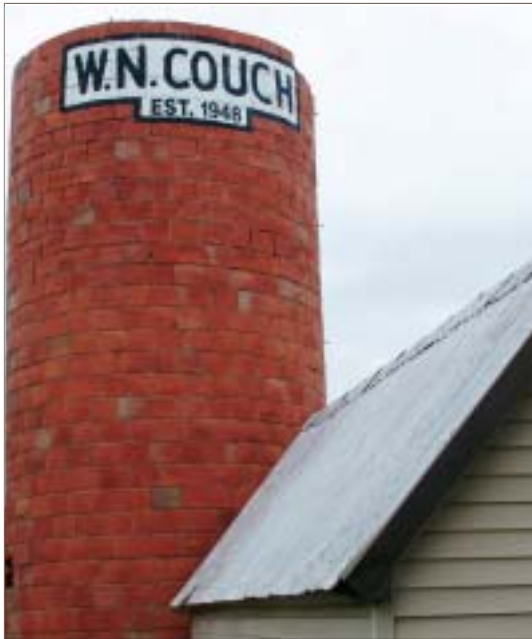
This silo sits at the edge of the W. N. Couch, Inc. compound in Tulsa, the site where founder Wilson Nolen Couch lived with his family when he started installing phone lines in 1948.
