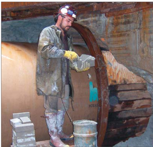
CCFRPM pipes were blocked in place to facilitate annular space grouting.
