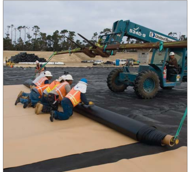
Workers roll out one of the 175 liner panels.
