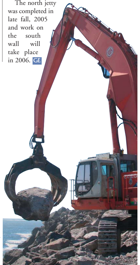
Fitting the excavator with a special front end package increased its lifting capacity.
