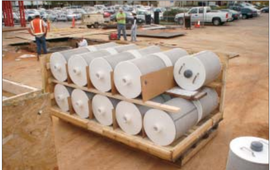
A crate of perlite-filled cylindrical cartridges sits ready for installation at the job site. Forty-two of these cartridges are placed within the media filtration device. Each measures about 18 in. by 22 in.
