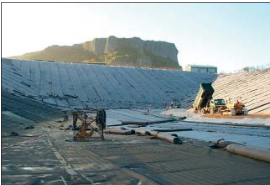
Landfill liner system is installed on the 12-acre waste management unit.
