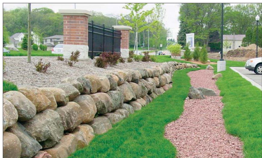
Trenches and soakaways, such as this infiltration trench in Wisconsin, are shallow trenches filled with rubble or stone to create temporary subsurface storage for infiltration of stormwater runoff; the runoff gradually exfiltrates through the bottom and/or sides of the trench into the subsoil and eventually reaches the water table.
