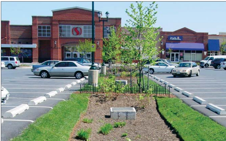
Frequently used in parking lots, bioretention systems such as this one in Maryland consist of a grass buffer strip, a sand bed, a ponding area, an organic or mulch layer, planting soil, and plants.
