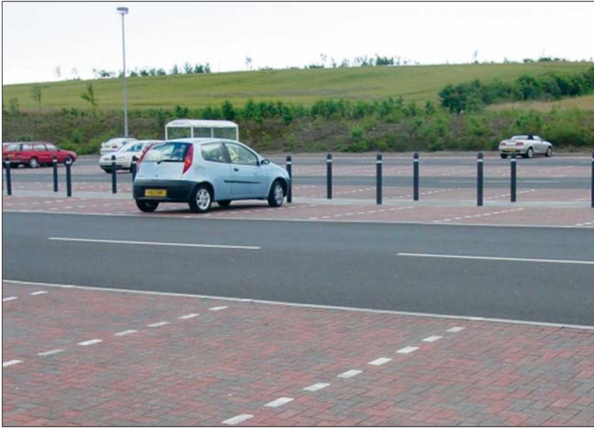
A porous pavement system, such as this one in Scotland, consists of a load-bearing, durable surface combined with an underlying layered structure that temporarily stores water before infiltration or drainage to a controlled outlet.
