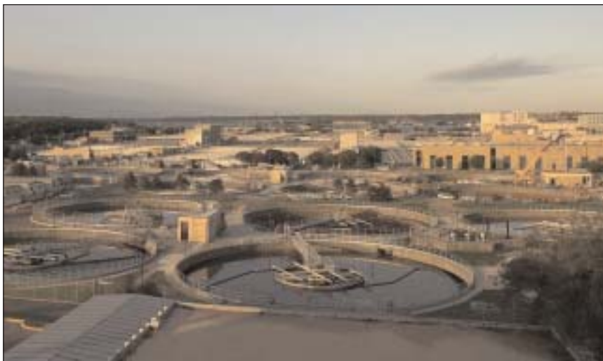
The Blue Plains WWTP in the District of Columbia has a capacity of 370 mgd, is a regional facility owned by the DC Water and Sewer Authority, and is the largest advanced wastewater treatment plant feeding into Chesapeake Bay.
