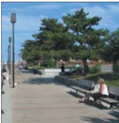
A single 3-in. by 8-in. by 16-ft plank of the new hardwood decking weighs between 300 and 350 lb.
