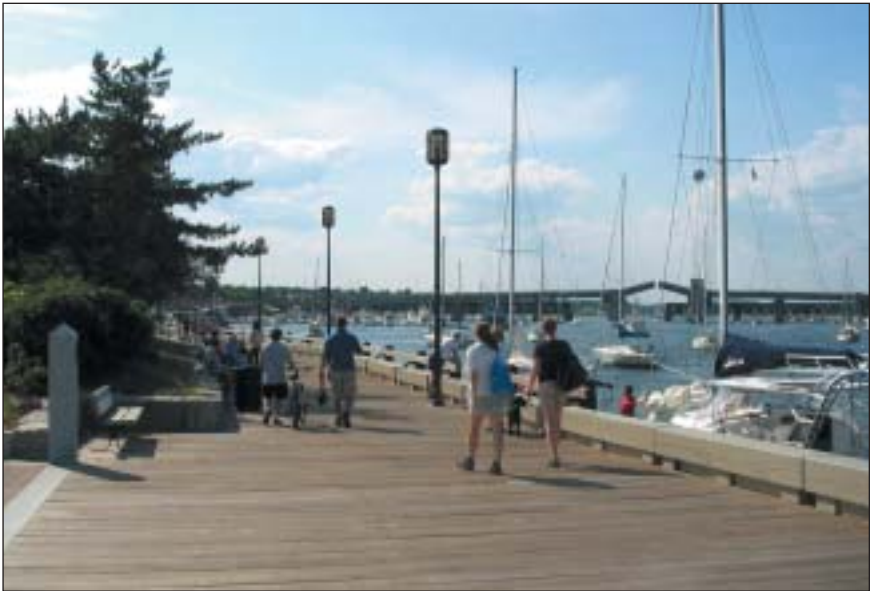
From the forests of Guyana all the way to Newburyport, MA, a durable tropical hardwood, Ipe, was used to re-deck the Peter J. Matthews Memorial Boardwalk.
