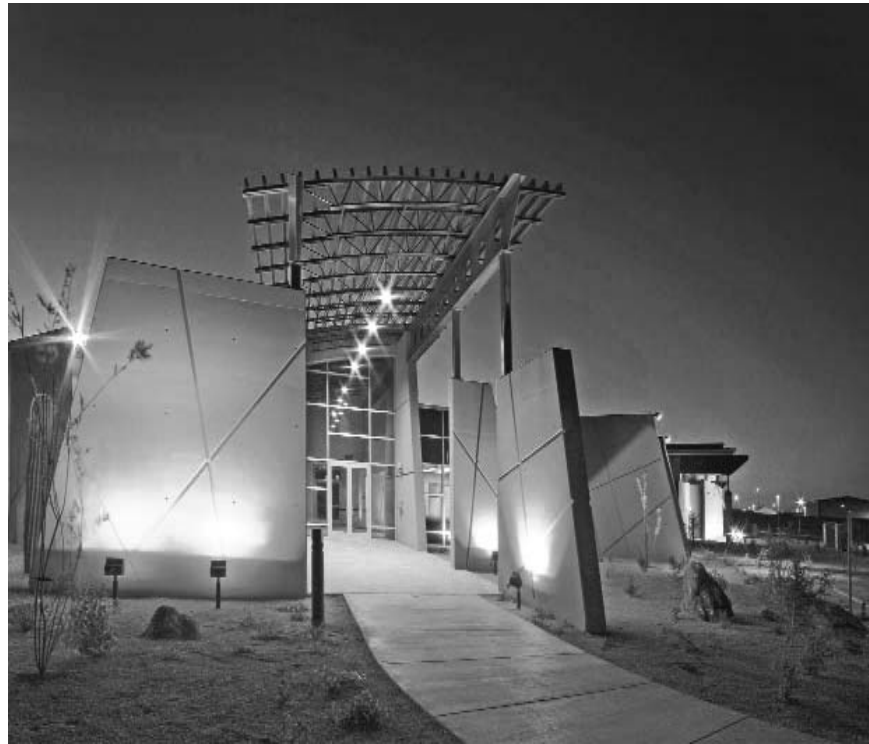
The award-winning Butler Drive Water Reclamation Facility in Peoria, AZ, produces high-quality effluent for aquifer recharge, allowing the city to earn water credits and therefore extract the equivalent amount of water from the aquifer to augment its supply and meet future needs. (Photo credit: Diego Ceja)
