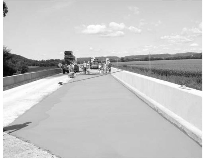
At left, the bridge maintenance crew waits for the mixing truck to arrive after using the Lightning Strike screed to prepare the bridge deck. At right, bridge maintenance crews use the screed while the cement is placed on the bridge deck.
