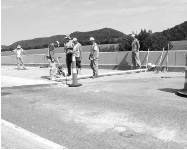
At left, the bridge maintenance crew waits for the mixing truck to arrive after using the Lightning Strike screed to prepare the bridge deck. At right, bridge maintenance crews use the screed while the cement is placed on the bridge deck.
