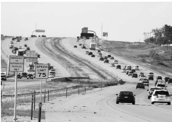
Completed construction showing variable message signs, cable safety barrier to avoid cross over accidents, and wider shoulders to allow for the HOV lane buffer.
