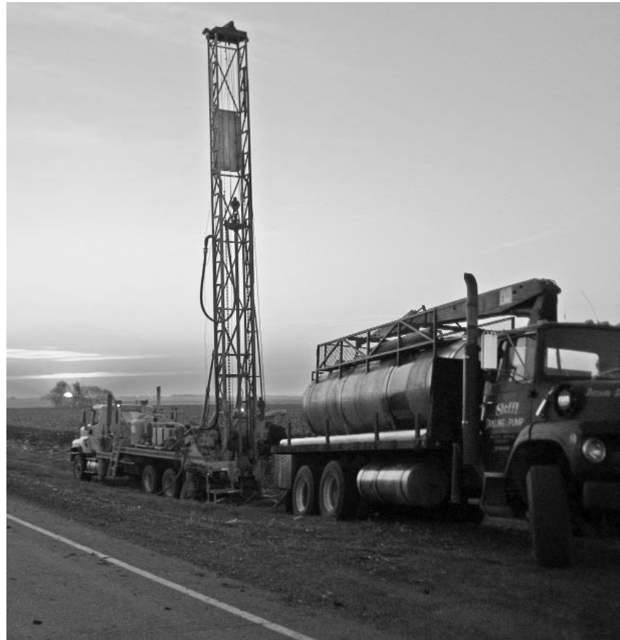
Test-hole drilling starts at a target site.
