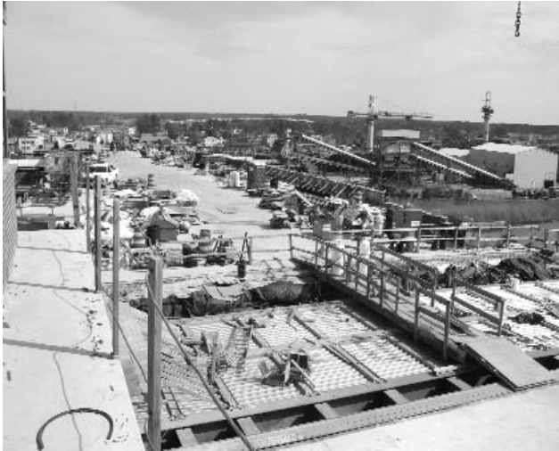
The Eltham Bridge project used innovative designs such as the bulb tee, a pre-stressed concrete girder that allows for longer bridge span lengths and reduces the number of piers needed in deep water.
