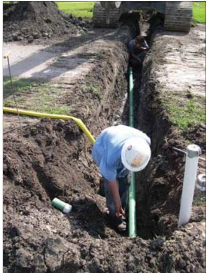
Vacuum sewer service lateral installation is simplified because lines are shallow and can easily be diverted over or under buried obstructions.
