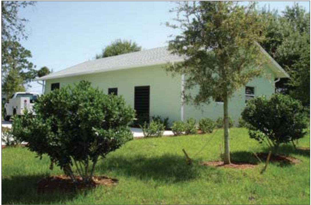
Single vacuum station, which services all of Rockridge's 400-plus houses, features an attractive stucco exterior that matches local architecture.
