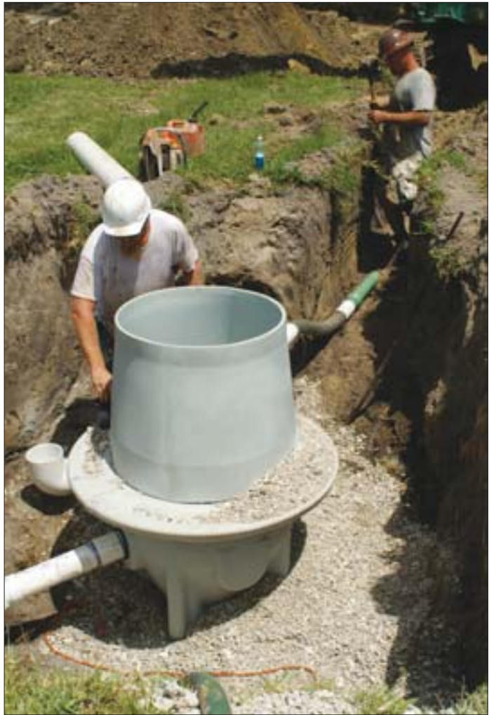
Shallow installation of vacuum sewer pits was important in Rockridge because the community is located on a layer of rock covered by sandy soil—making deep excavation costly—and in addition, groundwater levels are high.
