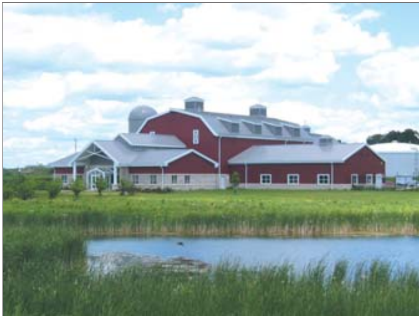
Geneva's new water treatment facility honors the local agricultural heritage of the area and provides open space, bike trails, and wetlands for the community. Photo credit: Black & Veatch
