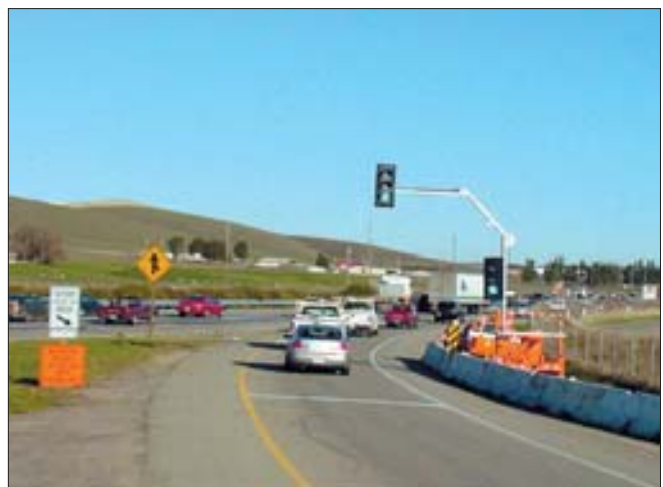
Portable traffic signals, which run on batteries and solar power, are easily moved from project to project and adjust to any slope.
