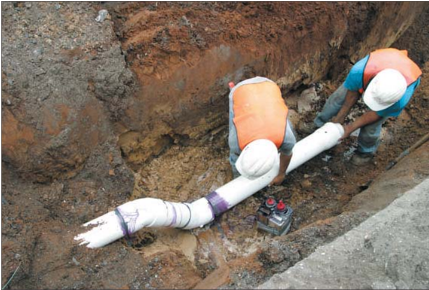
Unlike conventional sewers, which require the force of gravity and a continual downward slope to transport the wastewater, vacuum sewers use a pressure differential and are installed in a saw-tooth fashion, resulting in much shallower trench depths.
