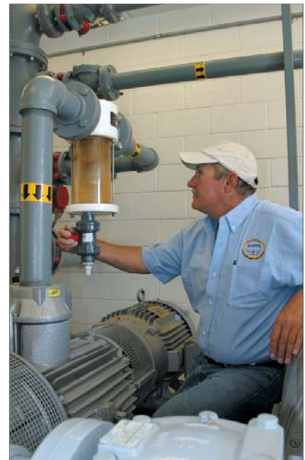
Vacuum stations are clean as well as operator friendly. Monitoring and maintenance are easy with a few gauges and charts checked daily and oil in the vacuum pumps changed regularly.
