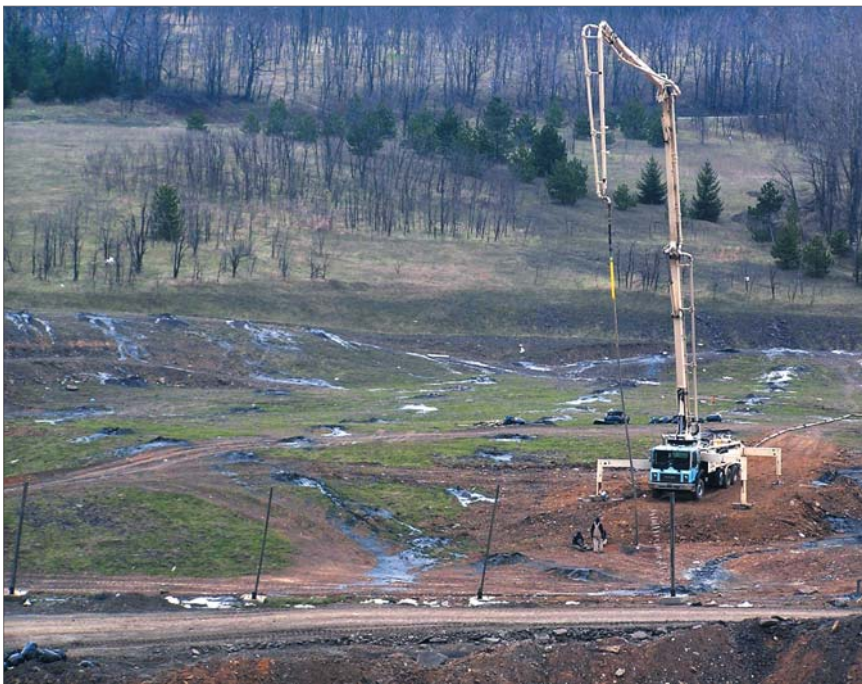
Panoramic view of grouting operations at Shade Landfill in Pennsylvania.
