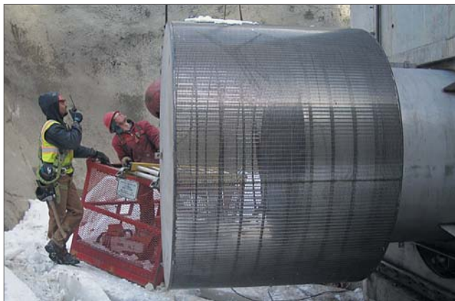
The intake tower features multiple gates that include unique screens for the protection of the fish.
