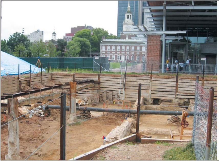
View of President's House excavation site on day of scanning. Three targets were set to capture the entire excavation area.
