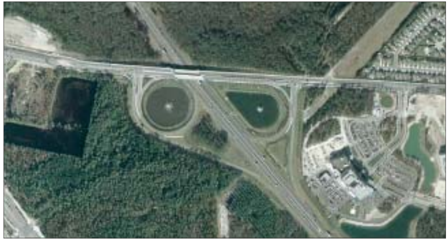
Two loop ramps, two diagonal ramps, tie-ins to the existing roadway, and two lanes of a bridge on St. Augustine Road were included in the interchange project.
