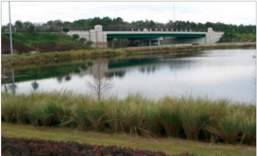
Built to Florida Department of Transportation standards, oversight was provided by the agency during construction.
