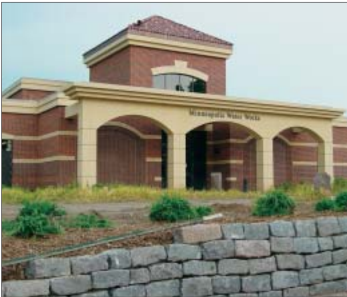
Membrane ultrafiltration was selected by the Minneapolis Water Works to remove pathogens like Cryptosporidium and Giardia from the potable water supply.
