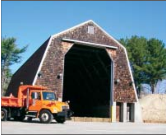
2005 award winning Plainfield salt storage facility.
