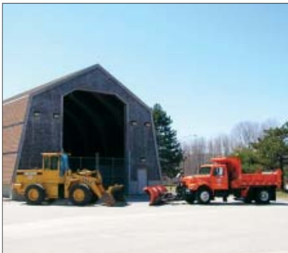
2005 award winning East Lyme satellite salt storage facility.
