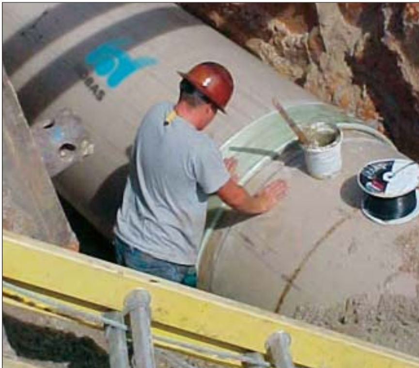
A vegetable-based lubricant helps make push-together assembly quick and easy.
