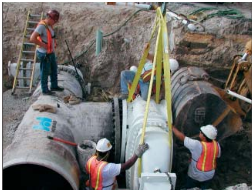
This T branch is one of a variety of custom manufactured fiberglass fittings that met the site-specific needs in Jacksonville.
