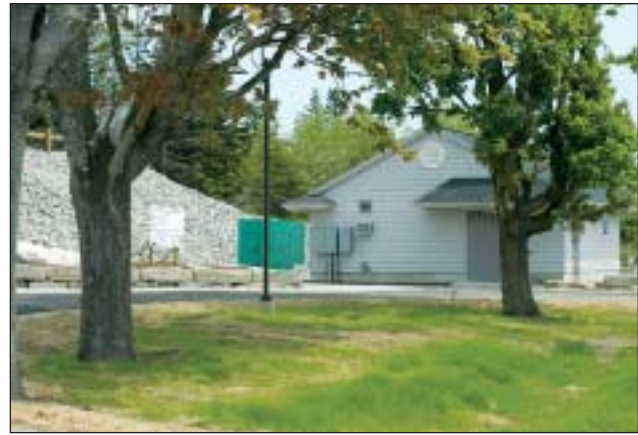
The facility employs ultra-violet disinfection, which eliminates the need to ship to and store chemicals on the island.
