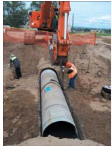
Sliplining pipe is lowered into the trench.
