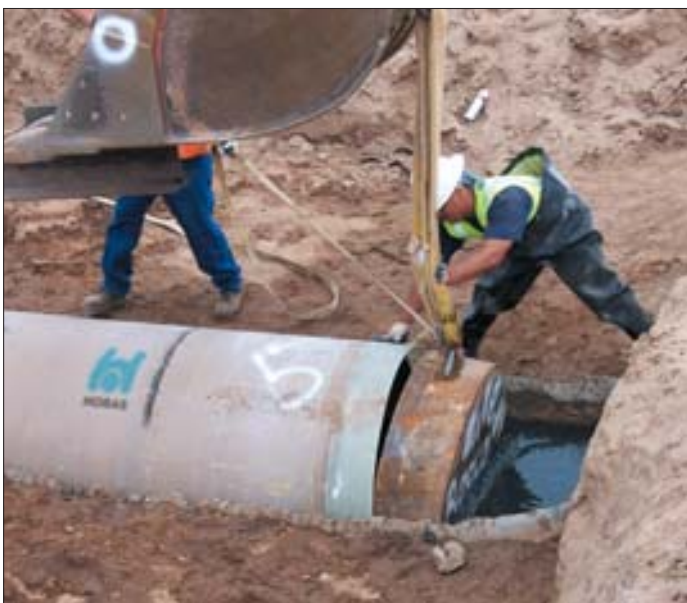
The push ring is placed on the pipe.
