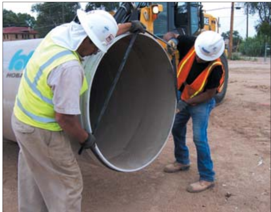
Gasket installation on the new pipe.
