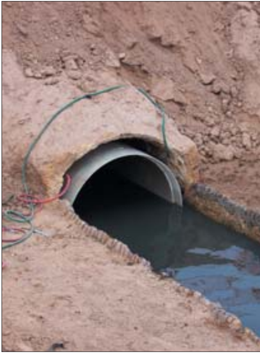
Note the tight fit of the new pipe.
