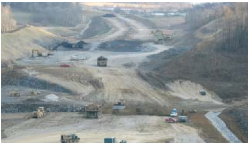
The scope of construction management and inspection services encompasses preconstruction plan review, scheduling and estimating, contract administration, construction inspection, CDS documentation, materials acceptance testing, project closeout, and public events coordination.
