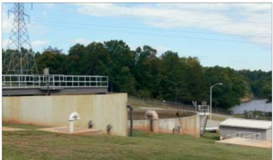
This is how the plant looked prior to the upgrade.
