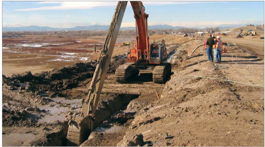
A gravel pit intended as a future water-storage reservoir was protected by a 1,350-ft long cutoff wall designed to separate the reservoir from groundwater.
